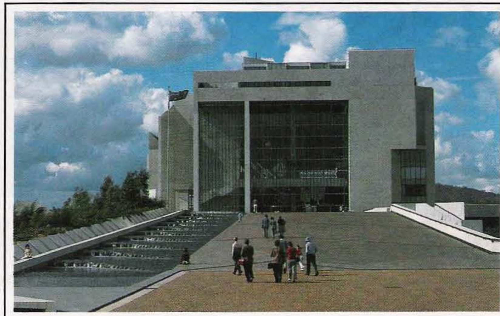
The High Court typifies the modern design of Canberra's newest buildings. The entry ramp is used for important ceremonies. (Photo by Robert C. Taylor)
