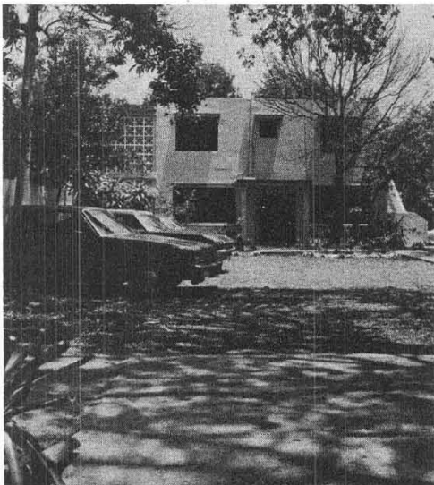
NEW OFFICE — The Caribbean Regional Office moved to new facilities in Santurce in metropolitan San Juan, Puerto Rico, in November, 1984. [Photo by Leroy Neff]
