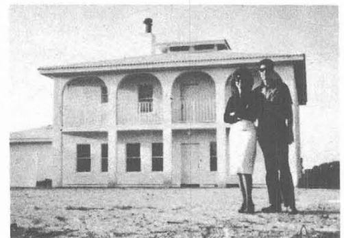
ENERGY SAVER — Danny and Mary Jane Nail pause in front of their house, which they designed and built. A state official said the residence was Florida's most energy efficient.
