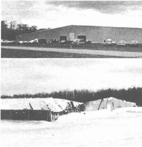
BEFORE AND AFTER — Members exit the repaired Church building in Mount Pocono, Pa., after 1981 Feast services, top photo. Above, the building following the January, 1978, storm. [Top photo by Michael Snyder]
