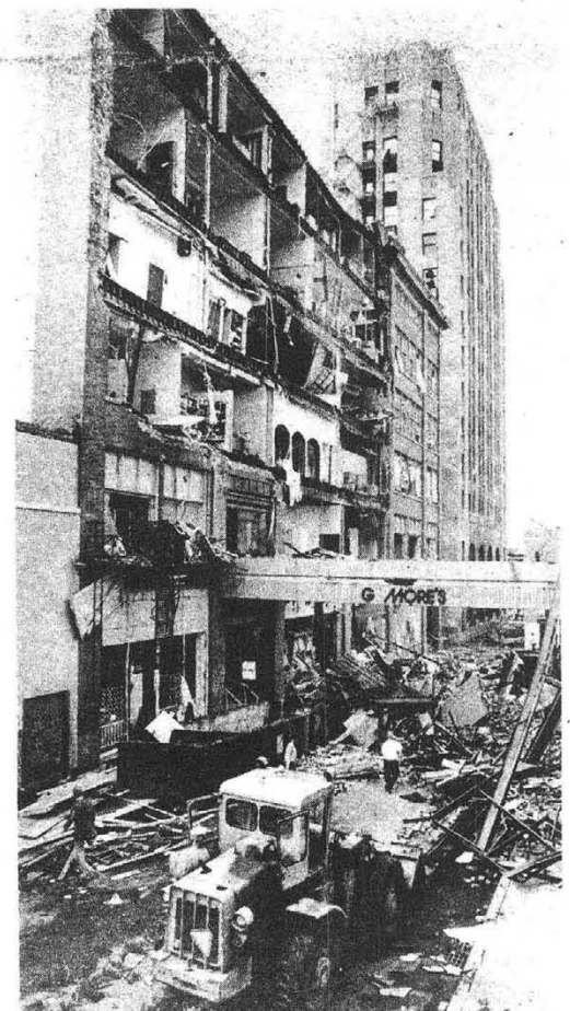
TORNADO AFTERMATH — Kalamazoo, Mich., residents begin cleanup following May 13 storms and tornado. Two persons died or injured outside the devastated department store as the winds ripped the wall onto the street. (Photo by Rick Campbell, courtesy of the Kalamazoo Gazette)
