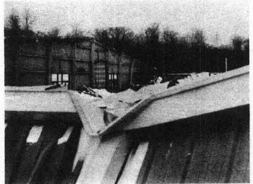
DISASTER — The roof of the Church-owned Festival building at Mount Pocono, Pa., collapsed under the weight of snow during a blizzard Jan. 28.
