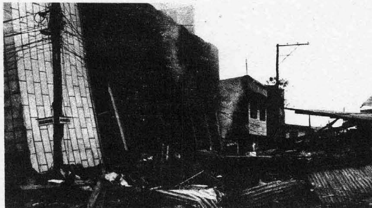
DEVASTATION — The earthquake that struck the island of Mindanao in the Philippines Aug. 16 destroyed many buildings, homes and lives, including what had been a gift shop and book center, above. Church members in the area escaped injury. [Photo by D'Exacto Studio, Cebu]
