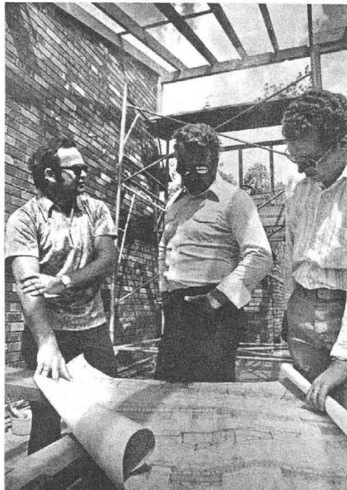
CHECKING IT OUT — Dennis Luker, left, shows International Division director Leslie McCullough, center, plans of the Australian Work's new office complex, which is under construction. Mr. McCullough toured the site during a recent visit to Australia. John Halford looks on. [Photo by John Robinson]
