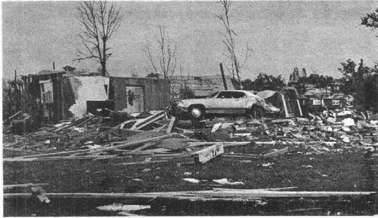
JONESBORO DISASTER — The wreckage shown above was a typical scene in the Arkansas city of Jonesboro after tornadoes swept through it May 27. These homes are only three blocks from the home of Mrs. Joyce Sparks, a member in the church. Notice the automobile where the living room used to be. [Photo by Williams Jacobs]
