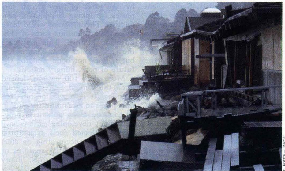
Beach residences collapse, Santa Cruz, California
