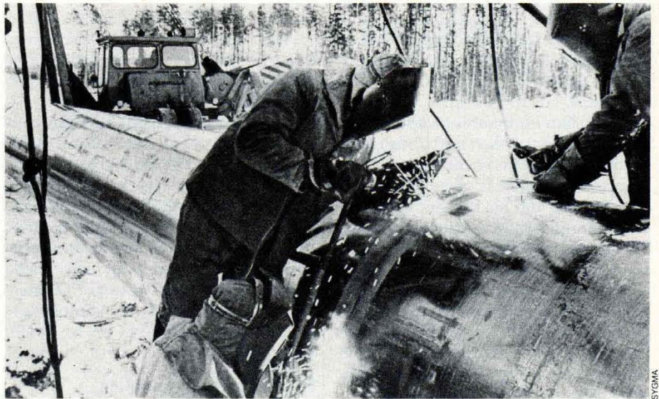
FOCUS OF CONTROVERSY: Workmen assemble pipeline in Siberia. Decision to purchase Soviet natural gas by Western Europe has angered American officials.
