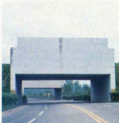
COLLAPSIBLE OVERPASS is designed to impede enemy wartime advance.
