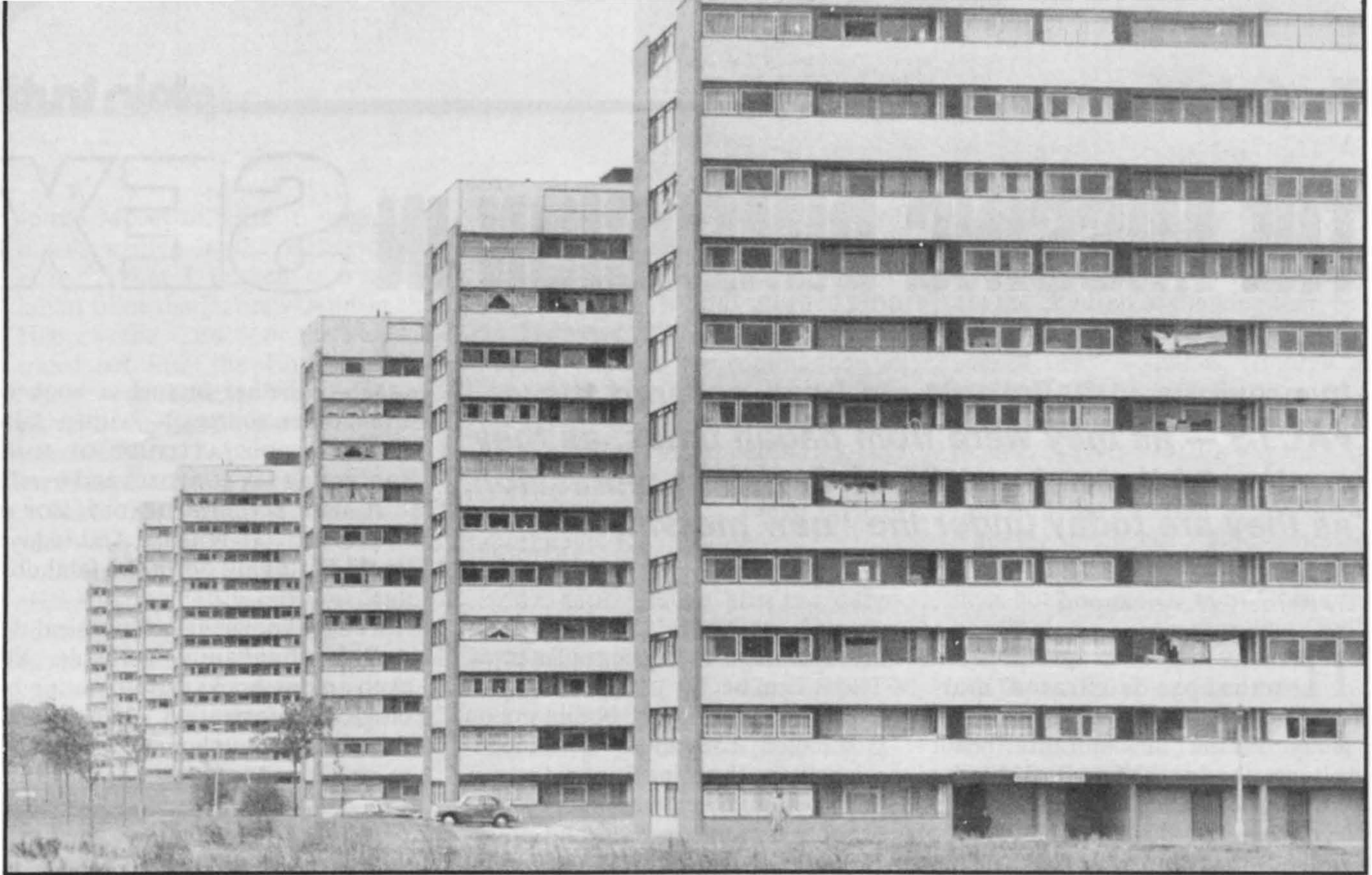
BIRMINGHAM is just one of many cities which has striven to solve its crippling housing problems by the construction of tower block estates.
