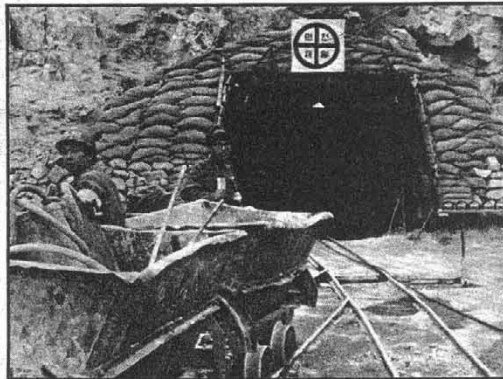
ENTRANCE to U.N.-dug intercept tunnel used to detect North Korean infiltration tunnels across Demilitarized Zone. Wide World
