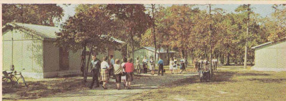
Temporary portable classroom buildings, of latest design, on Texas campus. To supersede them are two new classroom buildings, on architects' drawing boards, to begin construction in 1967.
