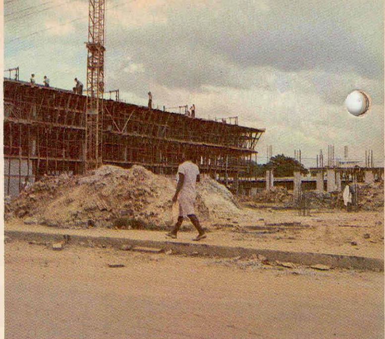
Government housing project, Panama City. One-quarter block away are wretched slums.
