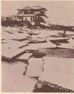
Right, Jacksonville, Florida — shattered pavement caused by hurricane Dora which struck in late 1964.
