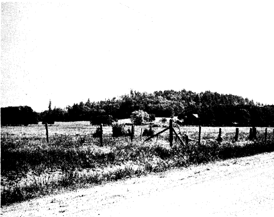
Site of Firbutte school where Mr. Armstrong held a six-weeks' campaign in 1933. The school was demolished several years ago when the Fern Ridge Dam was constructed.
