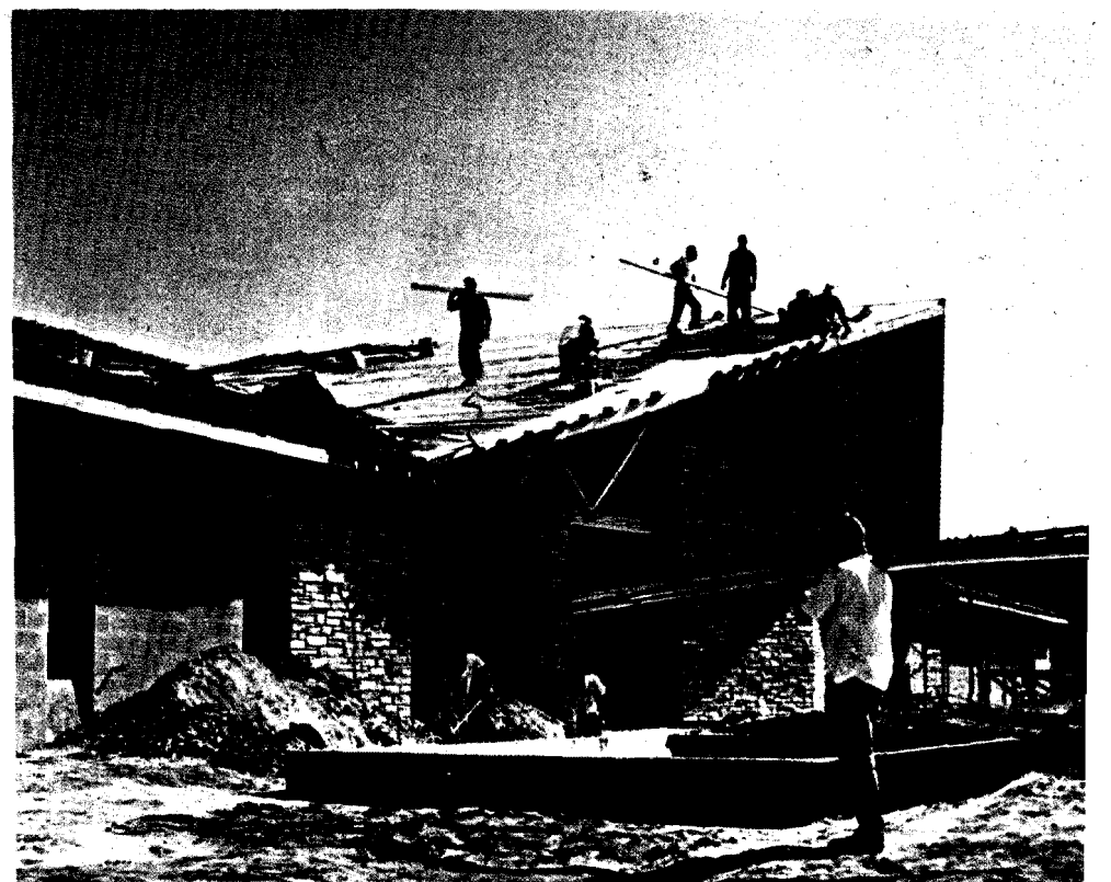
New administration building at the Big Sandy Festival site is shown nearing completion. Final touches are now being applied.
