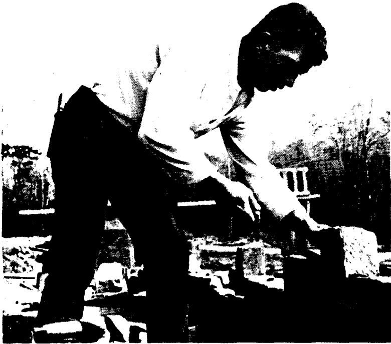
Here a craftsman lays some of the colorful exterior brick work characteristic of all the beautiful Administration buildings at the Feast sites.
