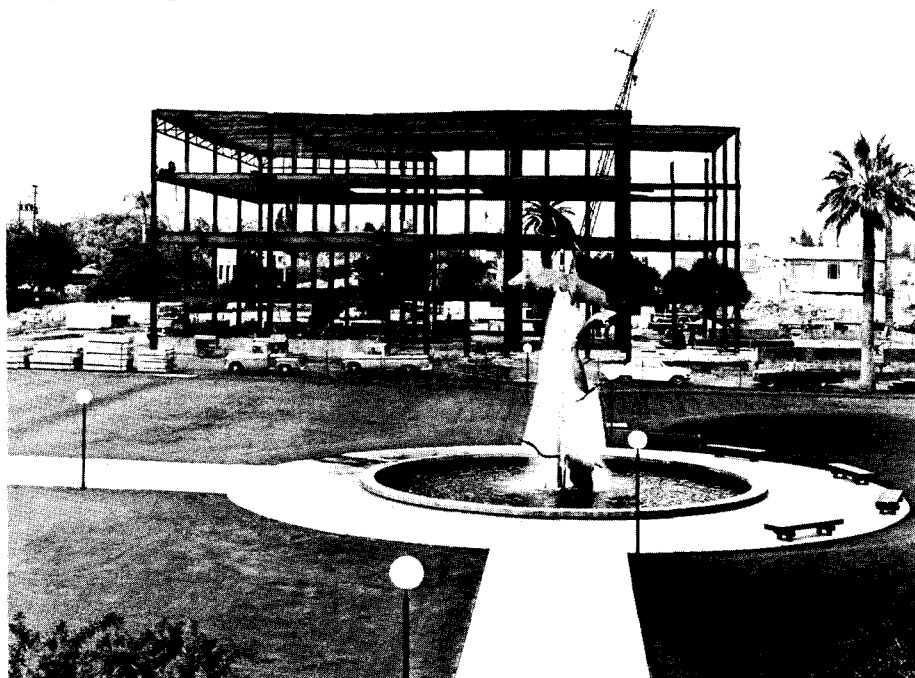
In February the steel girders were raised and in a few days the skeleton of the building began to take shape.
