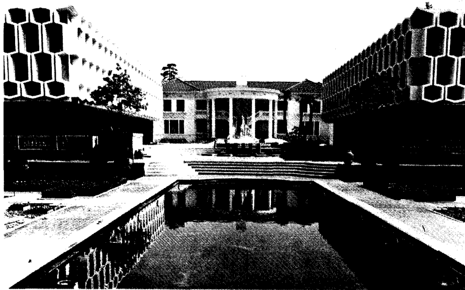
The Loma D. Armstrong Academic Center with its reflection in the sunken Italian garden pool.
