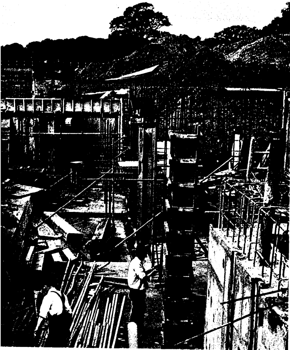
ABOVE—In the latter stages of construction the gymnasium begins to take shape. Notice the McAlpine construction firm's sign beside the scaffolding at the right. LEFT—Huge crane lifts steel girder cross beam toward its position in gym roof. CENTER—Complicated network of reinforcing steel rods insure structural strength—a factor unseen in the finished building.
