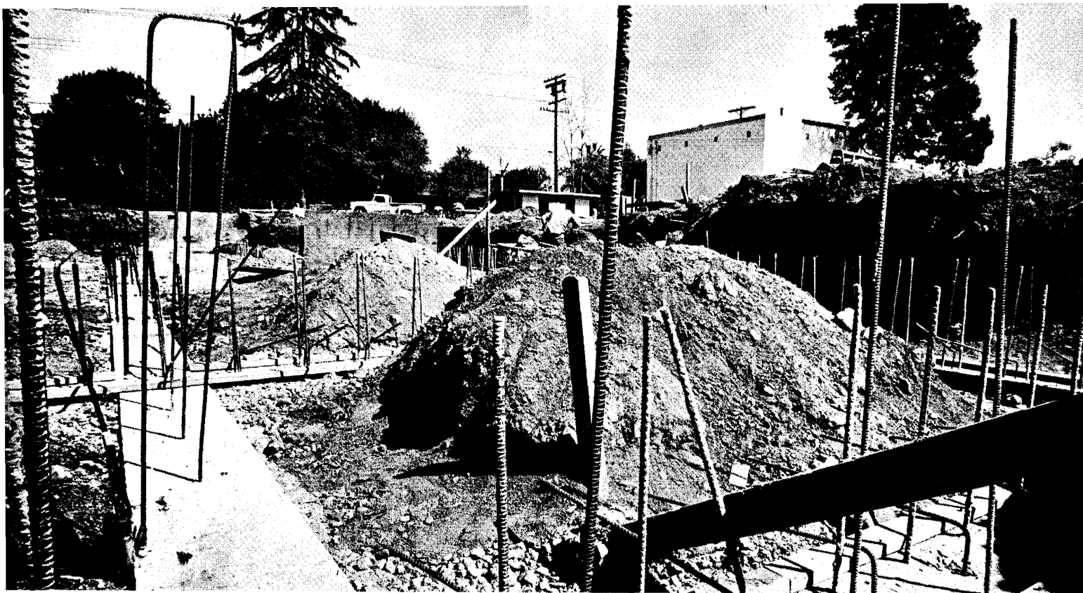
New gymnasium construction progresses rapidly.
