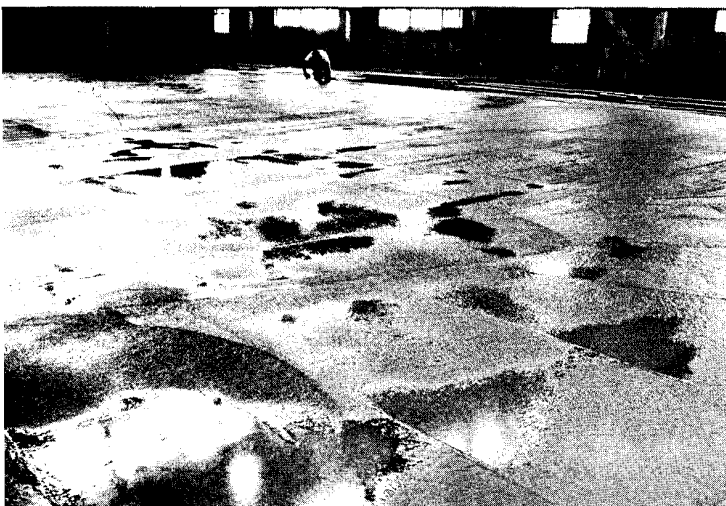
New concrete floor for new Press Building. Ambassador College Photo
