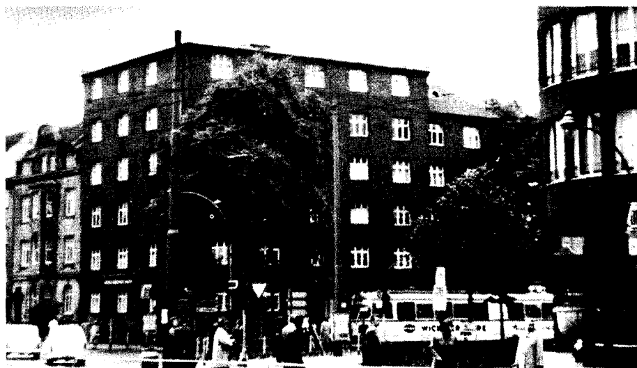
First glimpse of the new German office located near the heart of Düsseldorf—center of industry, finance, culture. Located on the third story is the 5-room office suite with room for expansion.
