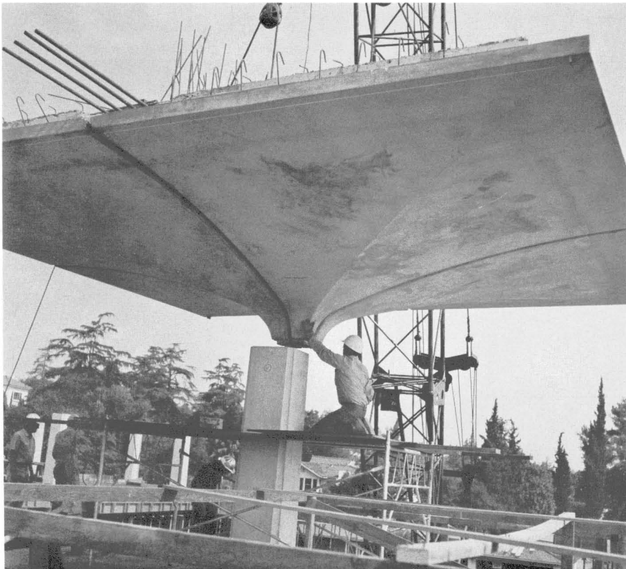
FIRST UMBRELLA —Huge crane very carefully lowers first Dining Hall umbrella into position while brave man directs its descent.
