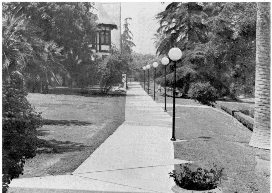
THE WALKWAY—The Construction Department is hurrying work on this beautiful walkway. The well-lighted and convenient promenade is just part of the changing Ambassador Campus.
