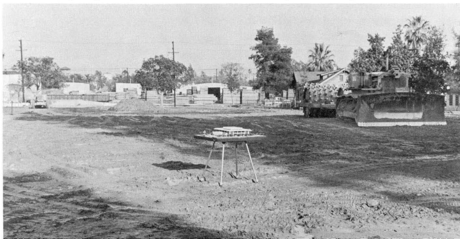
BELOW —Scale model stands alone in middle of Dining Hall building site.
