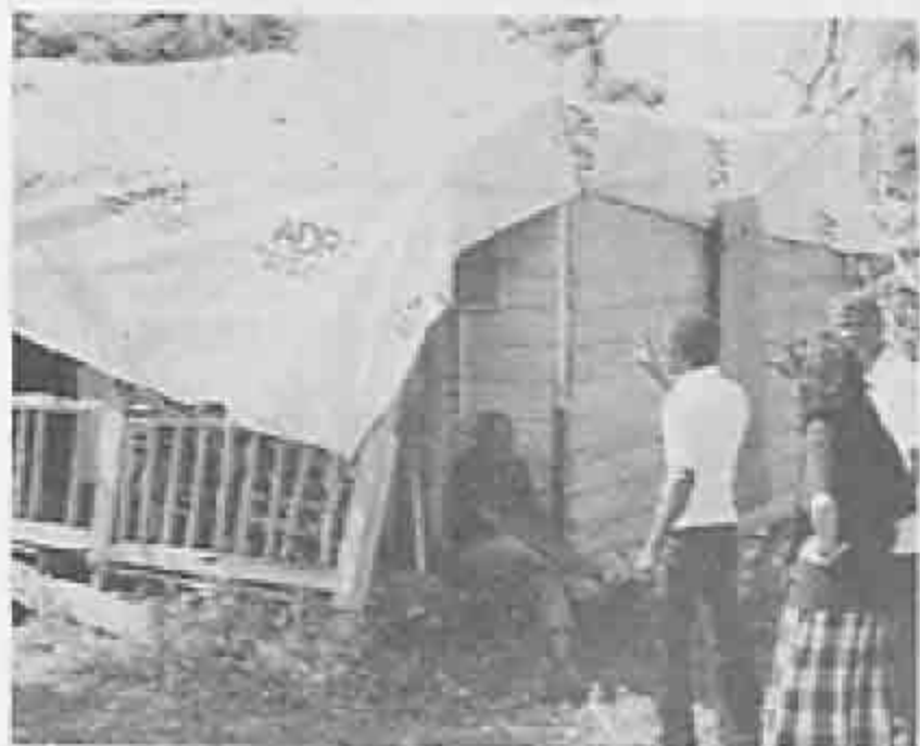
An ADRA tarp temporarily protecting a home that will need complete rebuilding.
