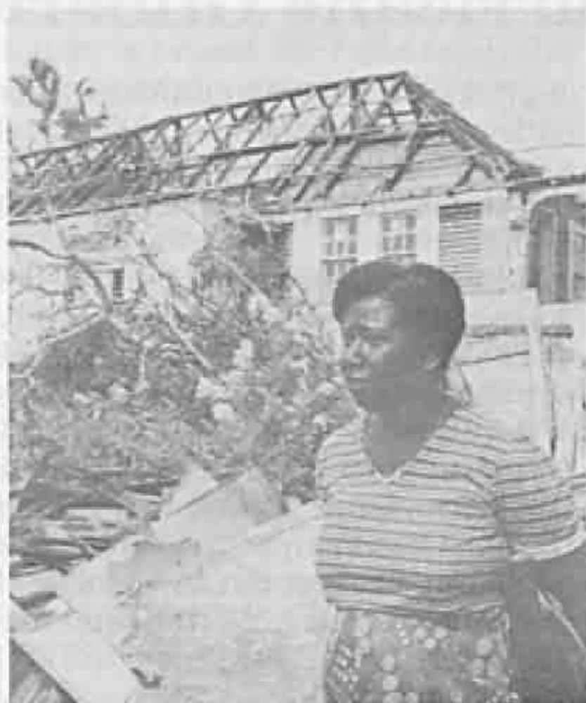
Typical storm damage to a home on the eastern end of the island.
